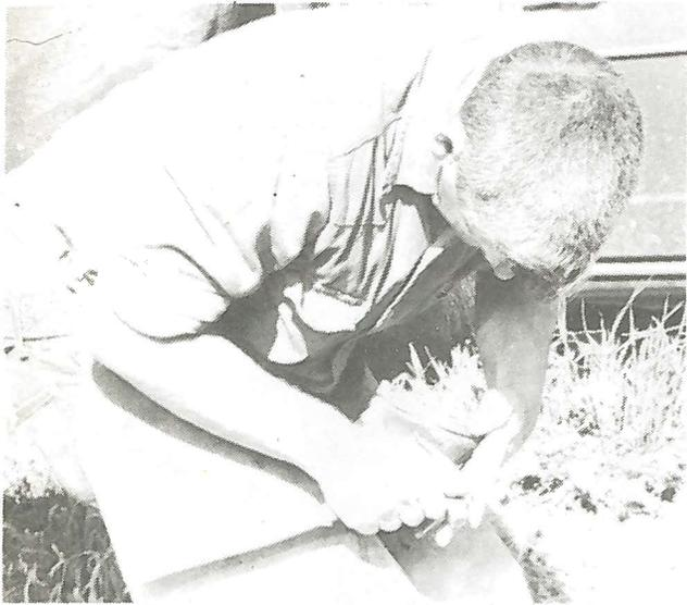
**A groove is rasped under the nails after they are twisted off. Then the end of the nails are clinched over into the groove.**
