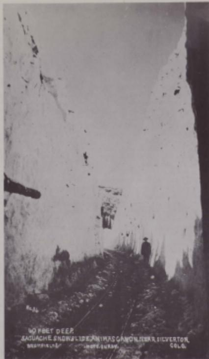
Figure 3. Cut in Saguache snowslide made to clear the Denver and Rio Grande Railroad tracks of avalanche debris. (Courtesy of the San Juan Historical Society)
