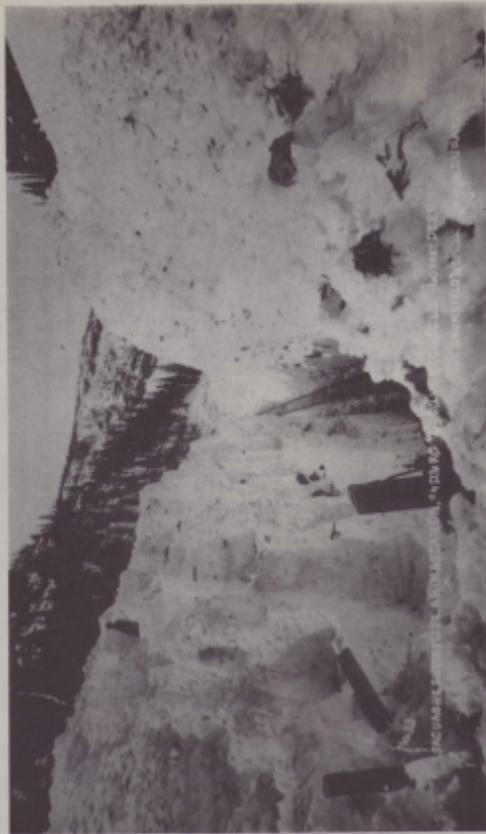
Figure 4. Cut in Saguache snowslide made to clear the Denver and Rio Grande Railroad tracks of avalanche debris. (Courtesy of the San Juan Historical Society)
